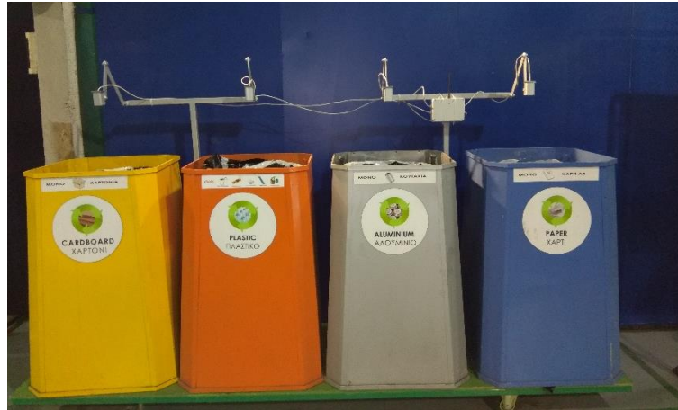
Figure 10: Fill sensors on set of recycle bins 1
