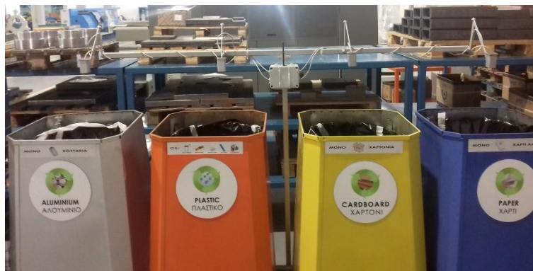
Figure 11: Fill sensors on set of recycle bins 2
